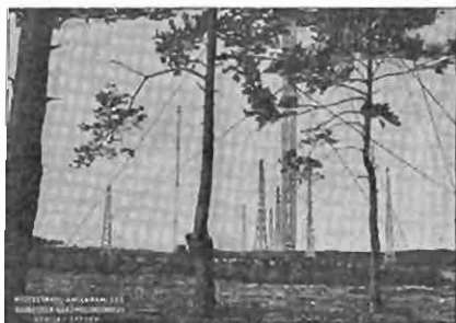
Here we have a glimpse of the Antennae system of "Deutschen Kurswellensenders" Station in Zeesen, Germany
